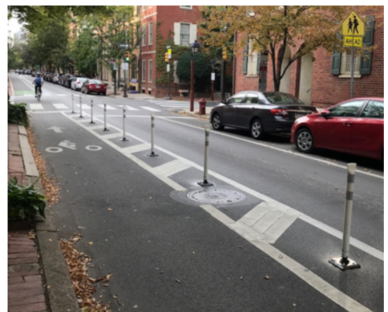
Bike lane delineators have been installed on Spruce and Pine Streets.
